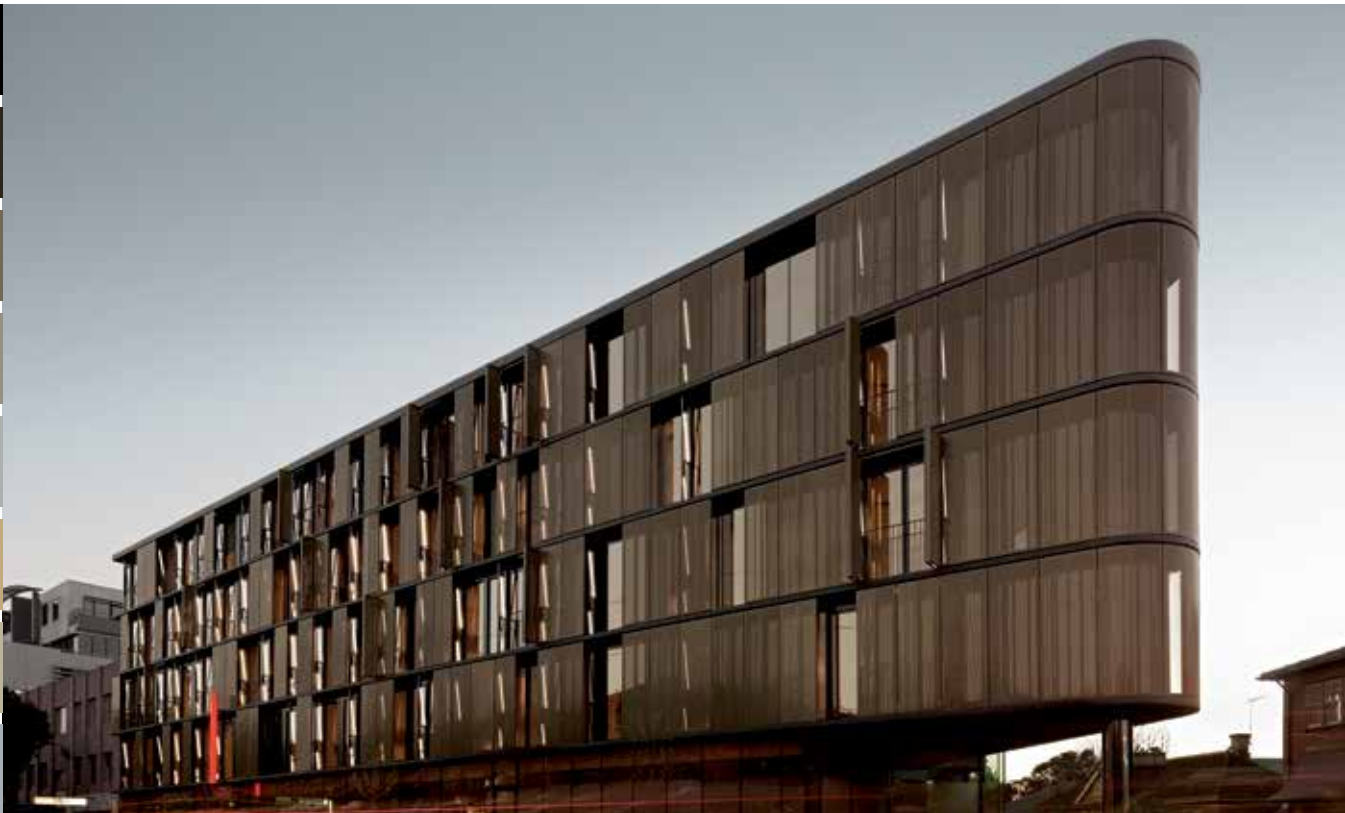
Mesh: ALU 6010, anodised in colour C33, project: Luna Apartments, Australia, architect: Elenberg Fraser
